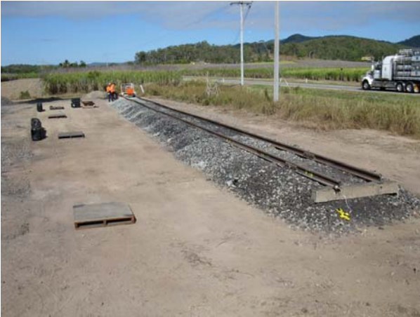
Figure 5 : GPR PVC calibration track panel
