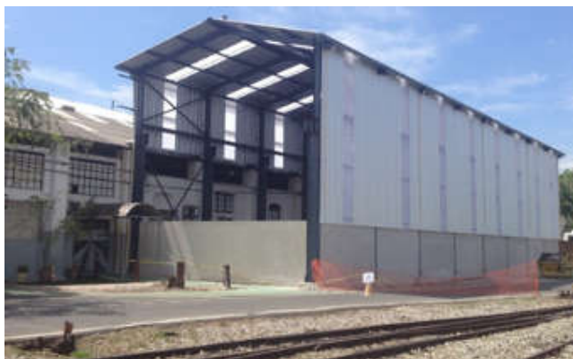
Figure 9. FCA's track vehicles workshop in Divinópolis-MG
